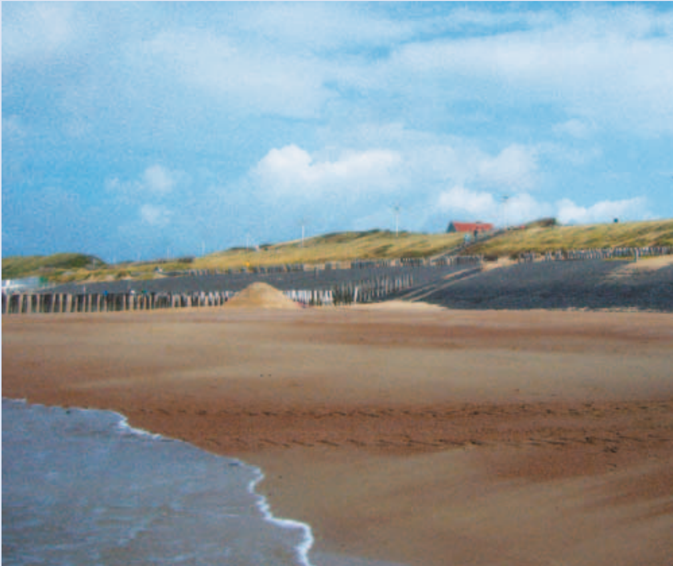
Image II-6. Dyke protecting settlement in Zeeland, Netherlands
